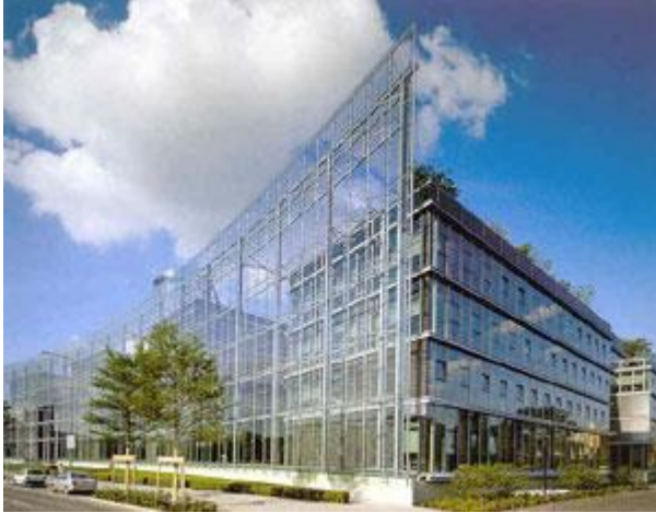
Figure 1.9. Some examples of noise barriers.
